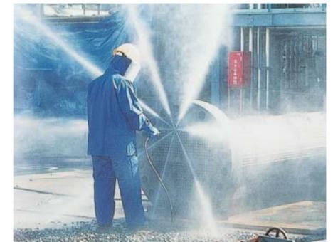
Cleaning of heat exchanger with Lance Nozzle.
